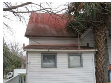
20 th Century Addition
