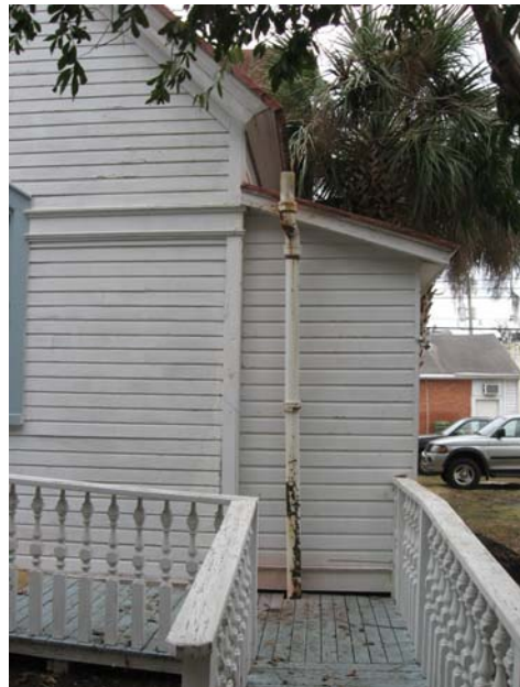
Restrooms sanitary exterior vent stack
