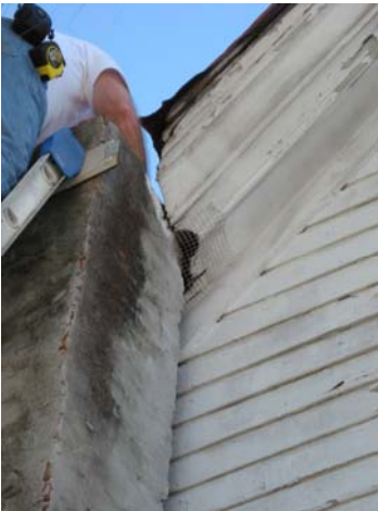
Deteriorated cornice
