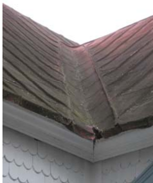
Open breaks in metal
