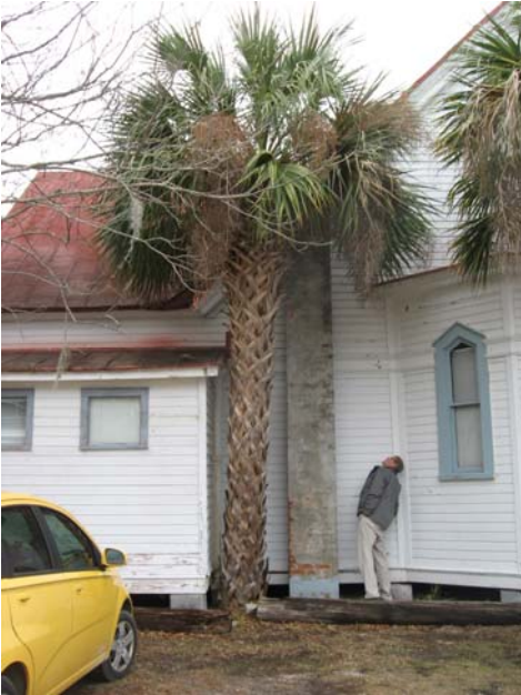
Palmetto tree canopy over chimney
