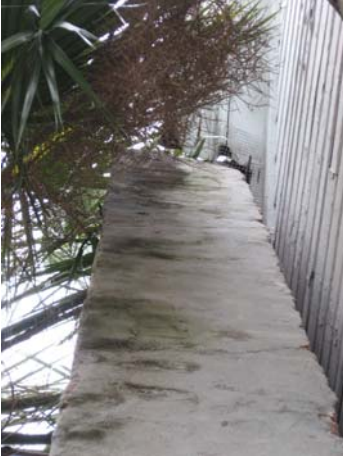
Free standing chimney
