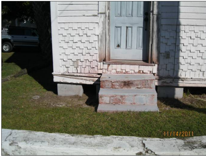
S-3 Door on right side
