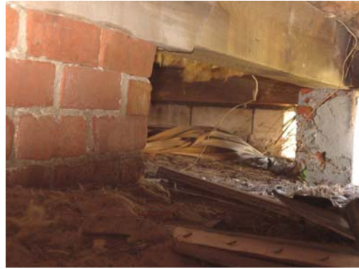
Masonry supporting pier
