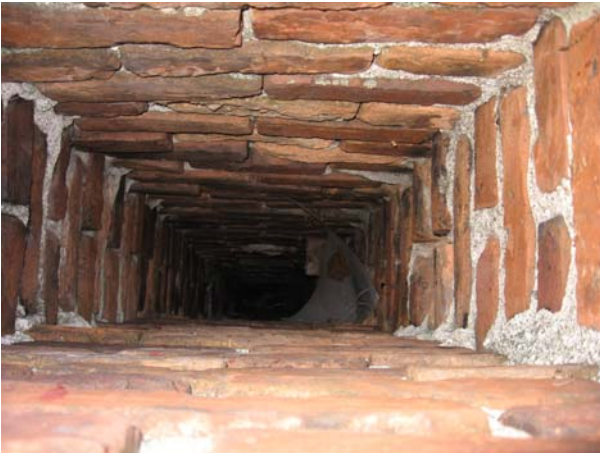
Open Chimney masonry flue
