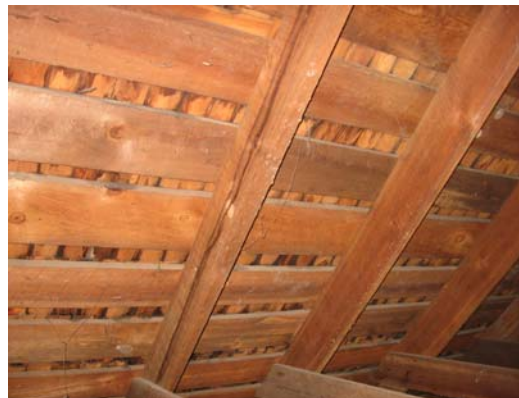
Open spacing to permit ventilation of shingles
