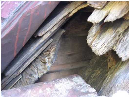
Edge condition at wood shingles under metal roof
