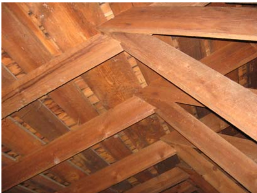
Attic sub-decking at roof ridge
