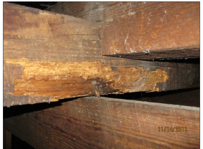
S-2 Horizontal member with insect damage
